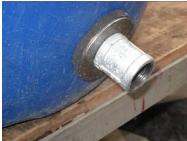
**Inner hot water tank: bulkhead fitting (outside the tank)**
